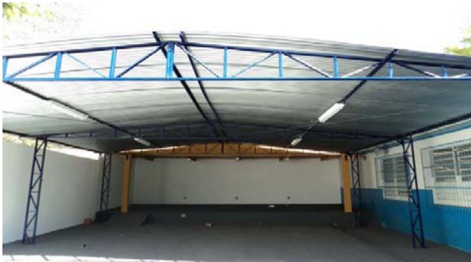
Fig1. Mini stage built at the school through a partnership between university, school, an NGO operating in the region and the private sector.
